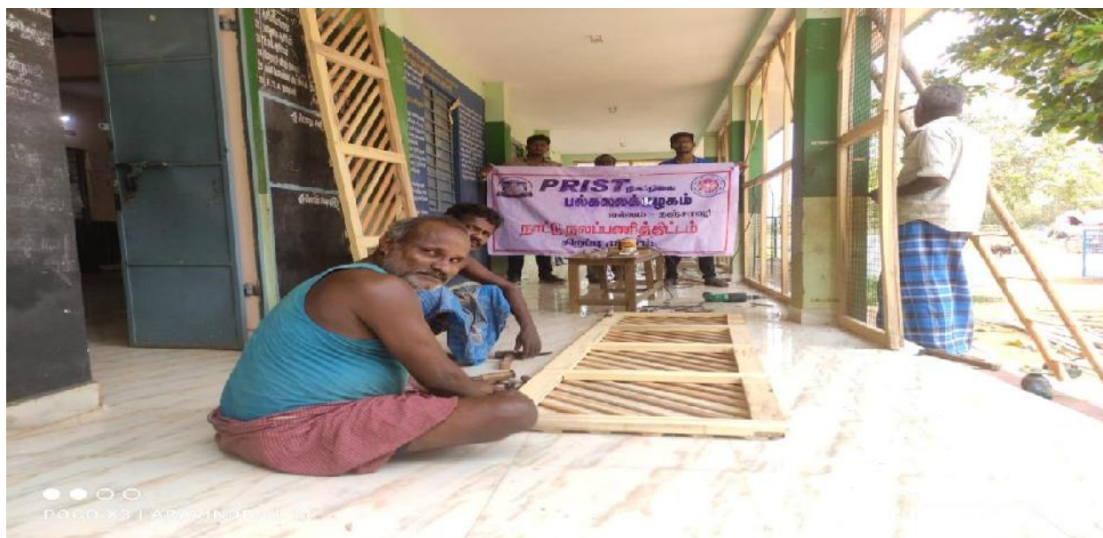
PRIST NSS in School renovation work at adopted village (Kuruvadipatti)
