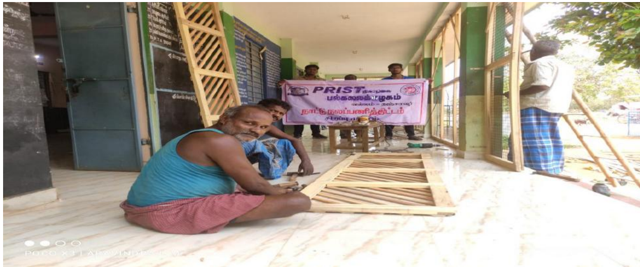
PRIST NSS in School renovation work at adopted village (Kuruvadipatti)
